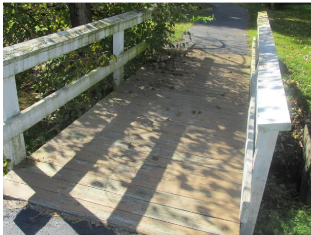
Bridge at Reynoldsburg
