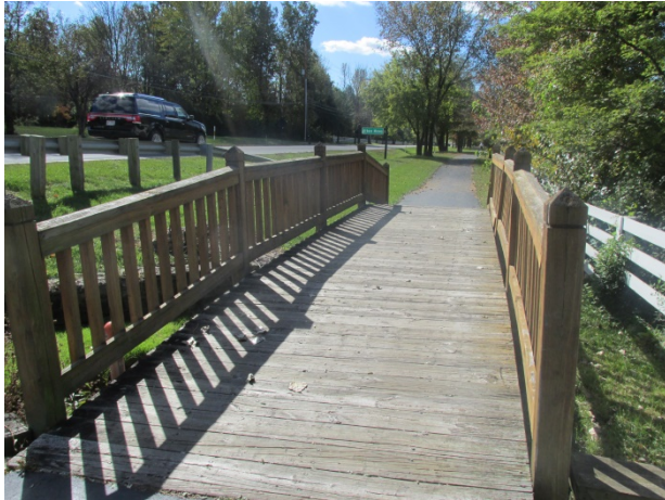
Bridge at Route 62
