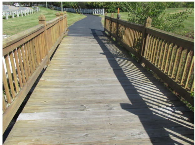
Bridge at Route 62
