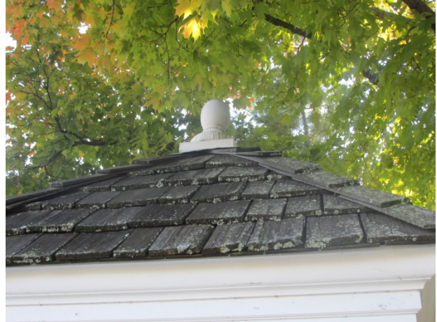
Wood shingle roof
