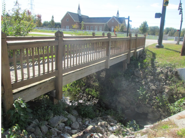
Bridge structure overview at Route 62
