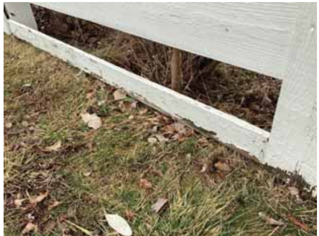
Finish deterioration
