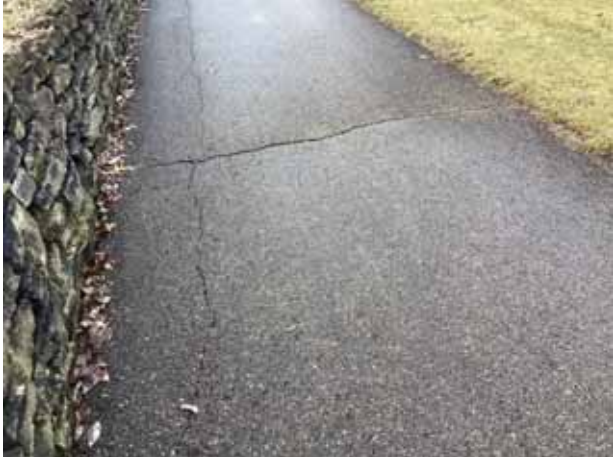
Pavement cracks
