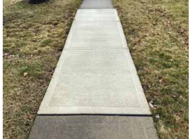
Recently replaced section
