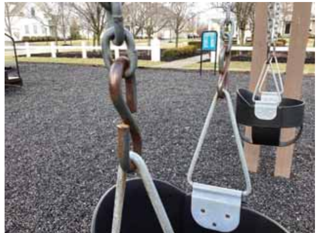
Rust at swings
