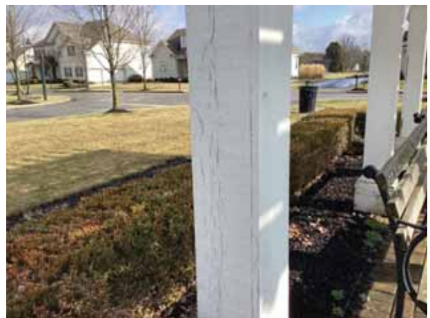
Finish cracks
