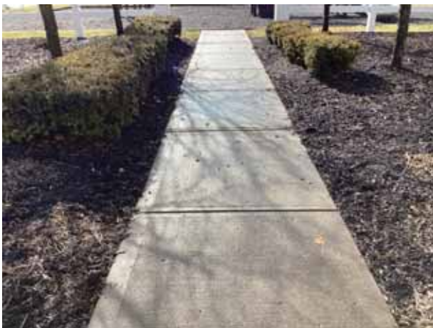
Concrete sidewalk at playground area
