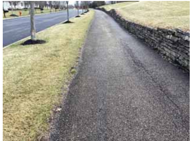
Asphalt pavement walking path overview
