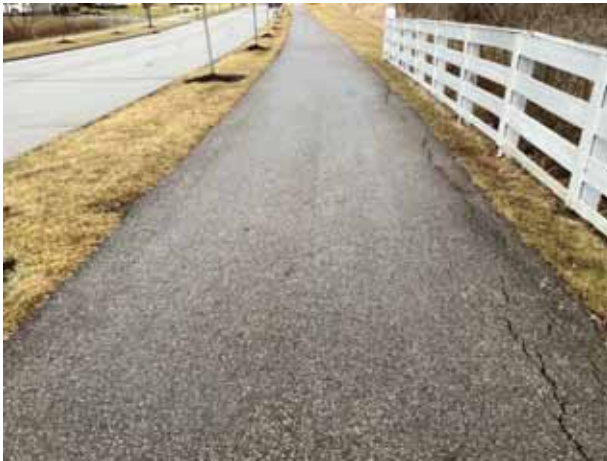
Asphalt pavement walking path overview
