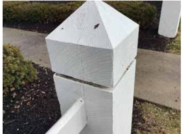
Finish crack
