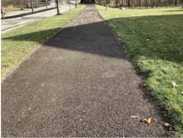
Asphalt pavement walking path overview
