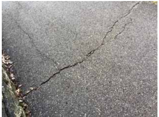
Pavement cracks
