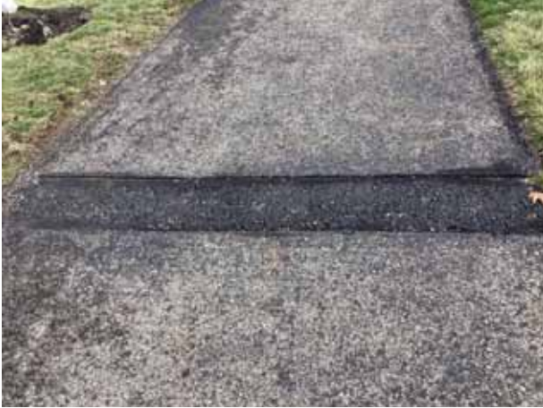
Previous patching repair
