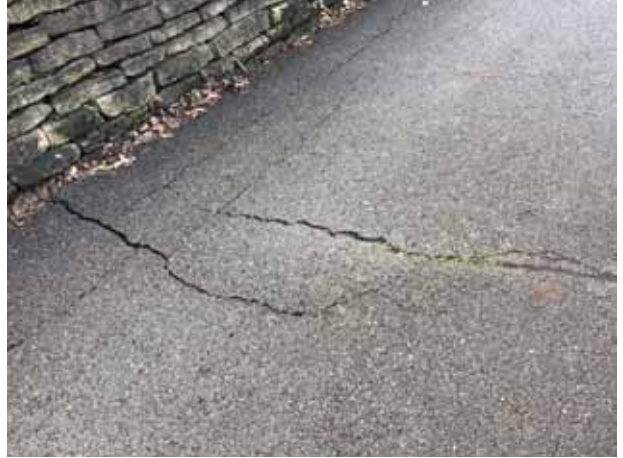
Pavement cracks
