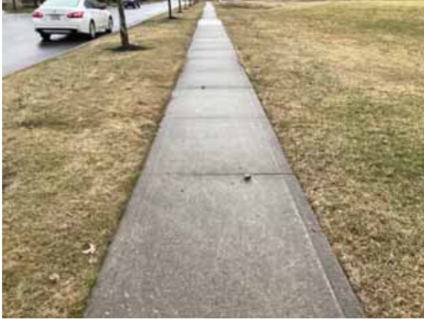
Concrete sidewalk overview
