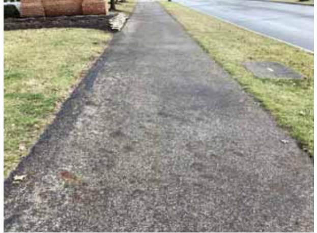
Asphalt pavement walking path overview
